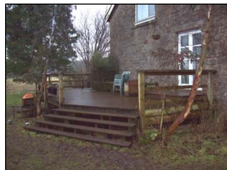
TIMBER DECKED AREA TO THE SIDE
